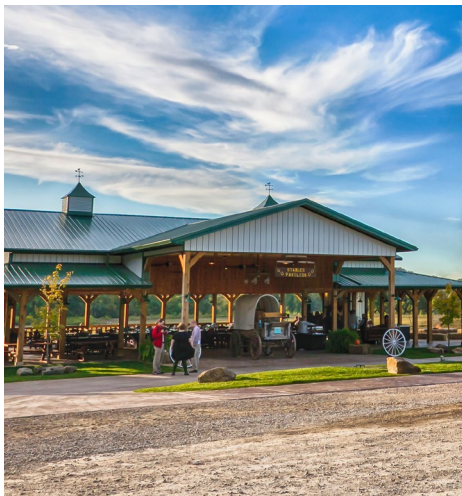
The Stable Pavilion
